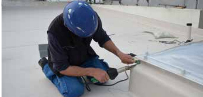
Detail work on the rooflight dome.
